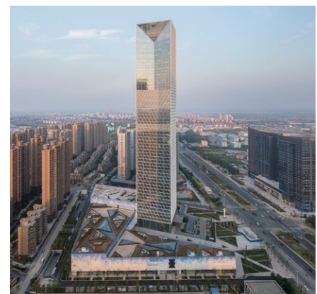
2015 Tallest #25: Jiangxi Nanchang Greenland Zifeng Tower, Nanchang, 268 meters © LV Heng-zhong
