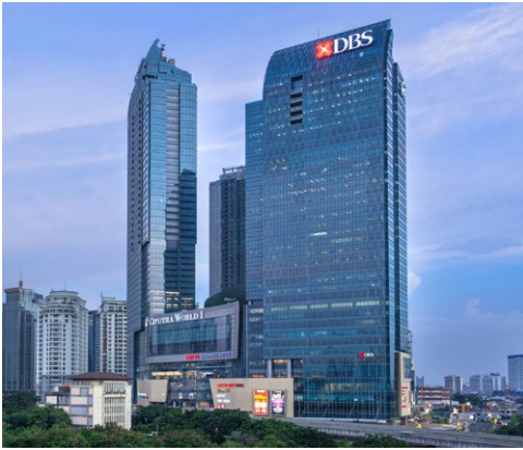
2015 Tallest #30: Raffles Hotel (with DBS Bank Tower), Jakarta, 253 meters © CallisonRTKL
