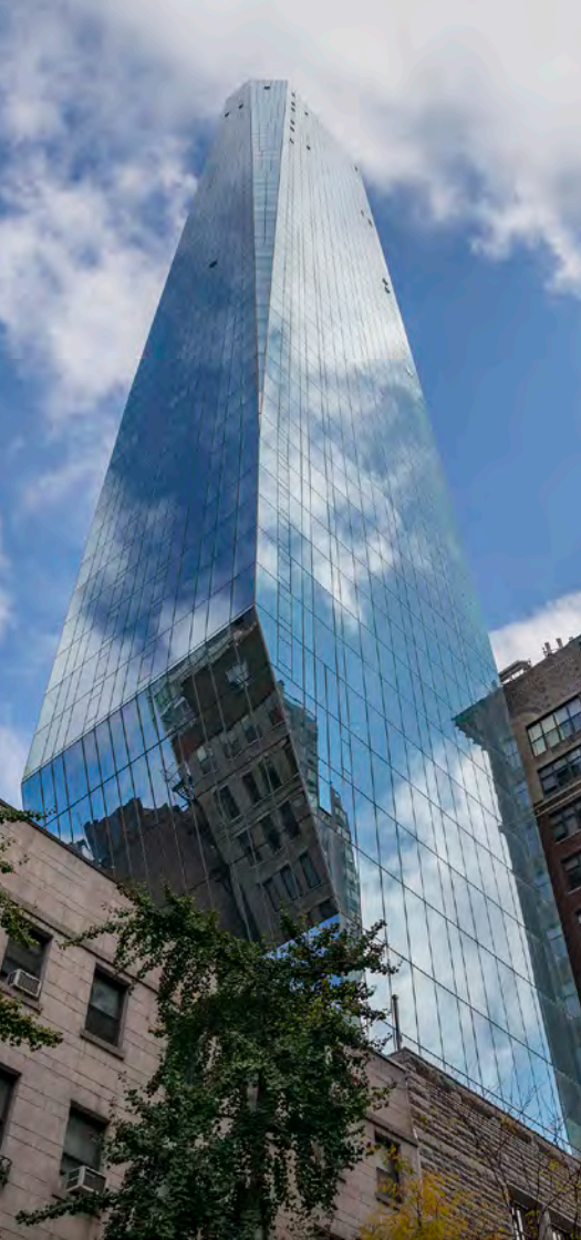
Figure 22. 62nd-Tallest in 2017: Madison Square Park Tower, New York City, 237 meters. © Lester Ali
