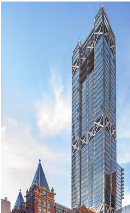
Figure 17. 111th-Tallest in 2017: The Beekman Hotel & Residences, New York City, 209 meters. © Lester Ali
