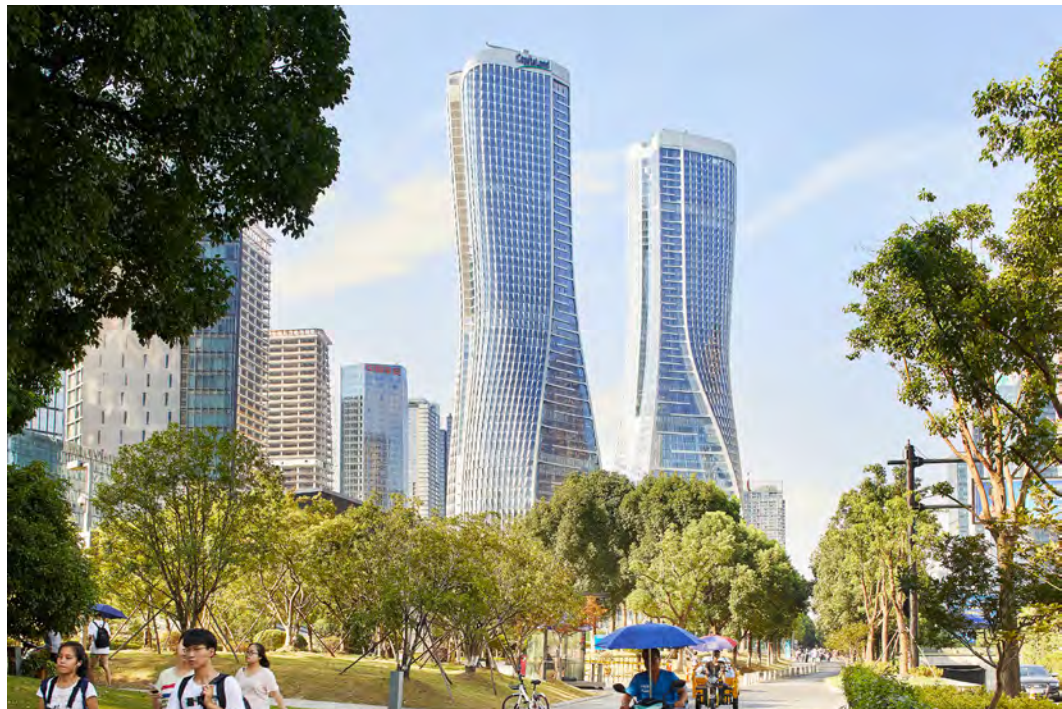
Figure 18. 35th-Tallest in 2017: Raffles City Hangzhou Tower 1, Hangzhou, 256 meters. © Hufton Crow
